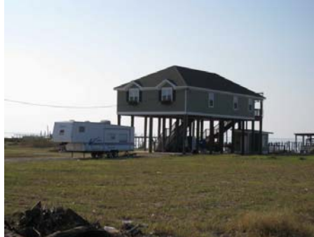
Housing being rebuilt in the Gulf Coast region following hurricane destruction.
